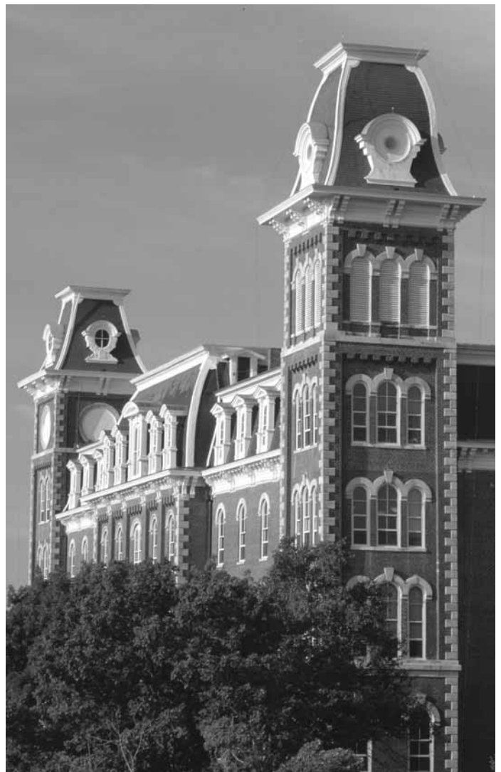
The original building of Arkansas' campus, Old Main, completed in 1876, symbolizes a connection to the past and the focus on the future, which presently come together at UA. Old Main was actually a copy of a building on the University of Illinois campus. The building at Illinois was eventually destroyed. Legend has it the only difference between the two buildings is the UA's north tower, which is higher than the south tower, which was symbolism for the Civil War since the lead engineer was a northern veteran.
